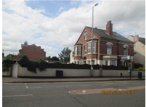
South east (front) elevation of site and main house
